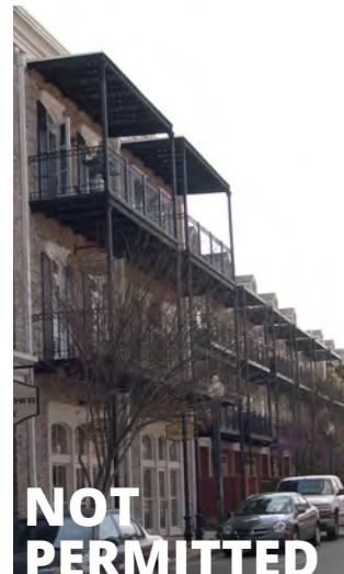
Balconies: Covers More than 40 Percent of Facade
