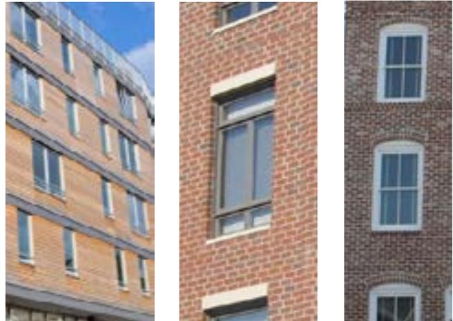
Figure 135-4.3-A. Vertically Oriented Windows with Expressed Lintels
